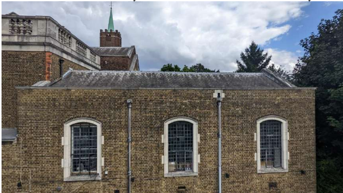
5.5 West Elevation Roof from Vicarage Roof
