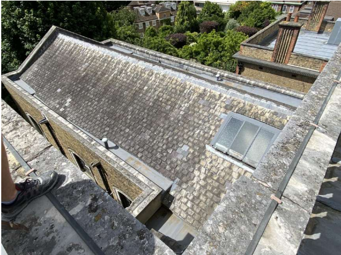
5.1 Choir Vestry Roof from Nave Roof
