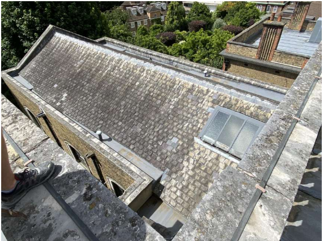
5.1 Choir Vestry Roof from Nave Roof
