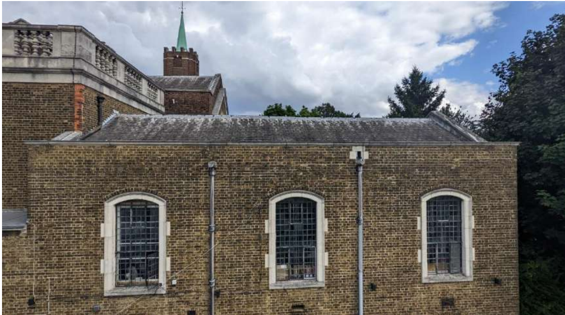
5.5 West Elevation Roof from Vicarage Roof
